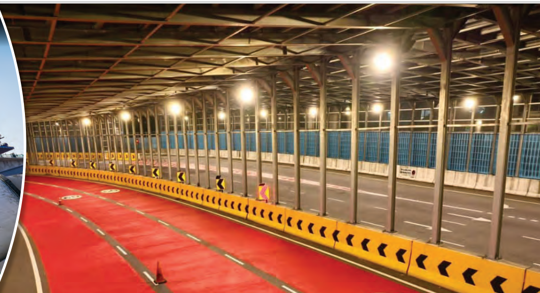
Installation of Geveko PlastiRoute™ High Skid Resistance Rollgrip at DASH to improve road safety measures.
