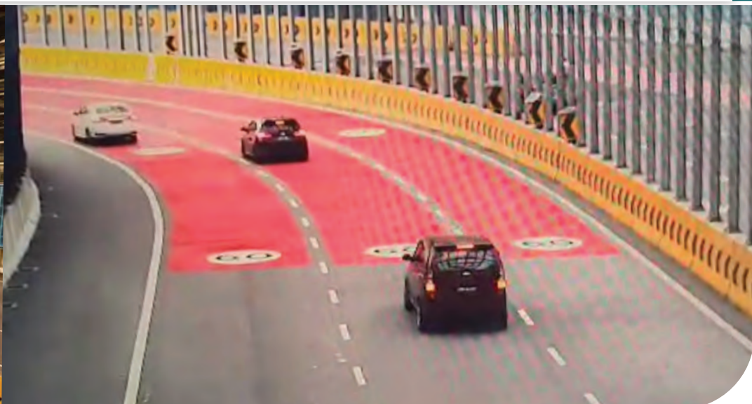
Installation of Geveko PlastiRoute™ High Skid Resistance Rollgrip at DASH to improve road safety measures.
